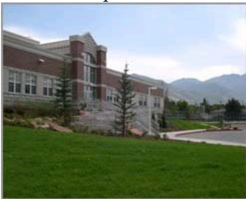
Dilworth Elementary – rebuild
