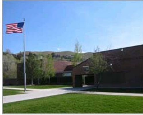
Ensign Elementary – retrofit & addition
